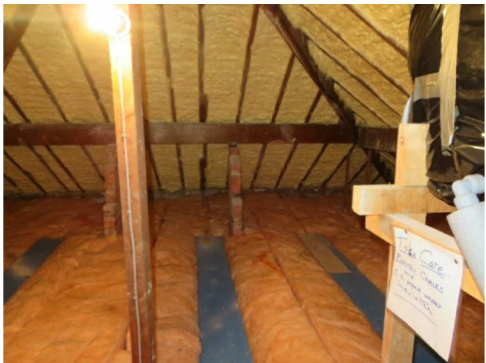
Spray foam between rafters
