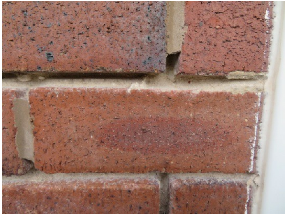
Eroded pointing
