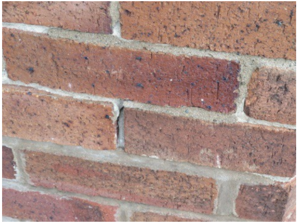
Eroded pointing
