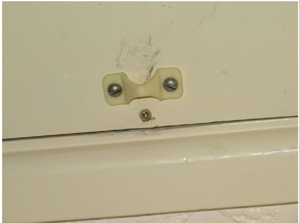
Screw holding loft hatch in place
