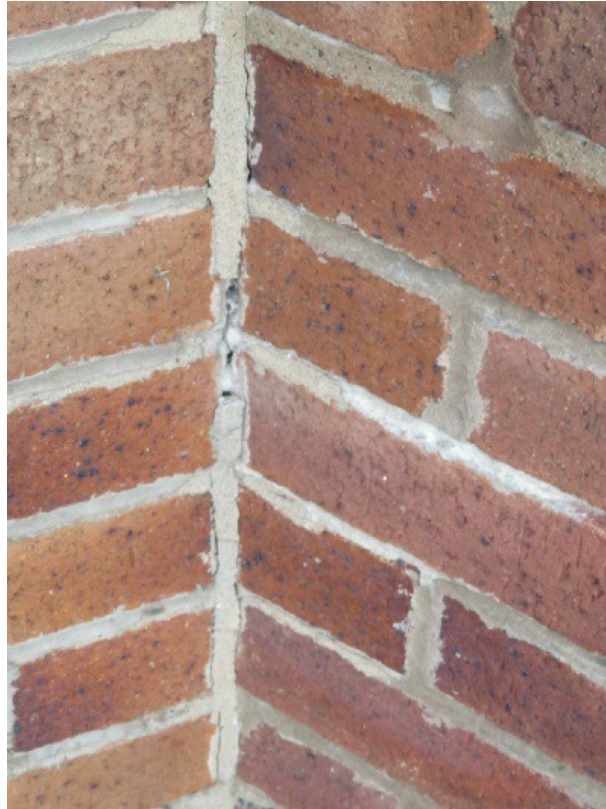
Eroded pointing
