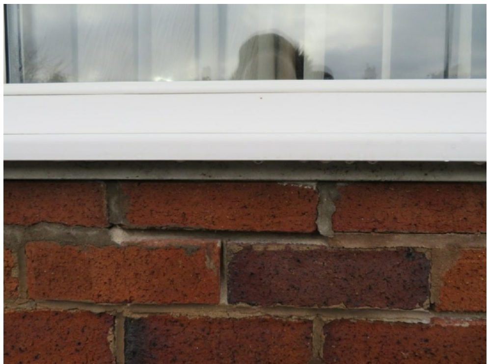
Eroded pointing
