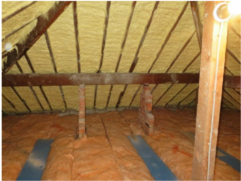
Spray foam between rafters
