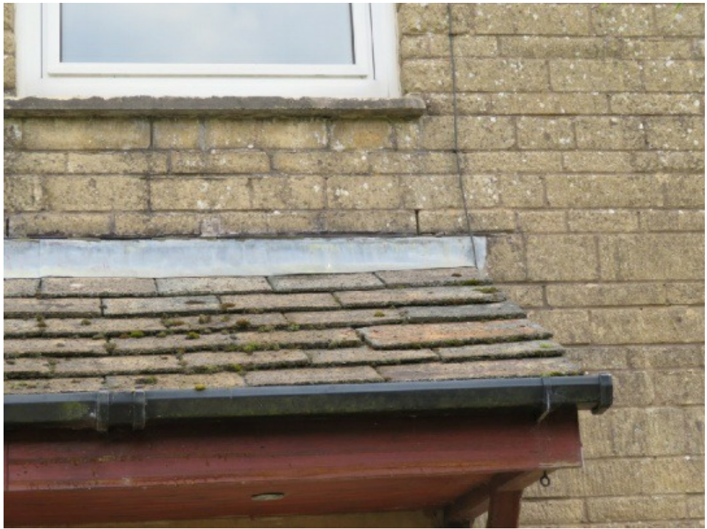
Eroded pointing
