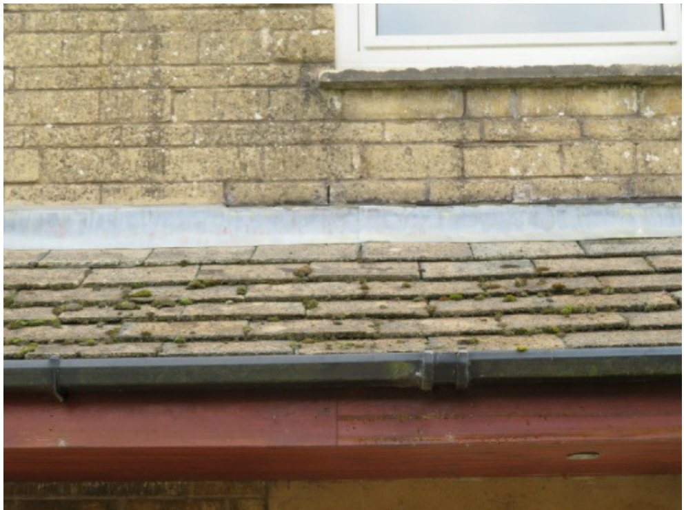
Eroded pointing
