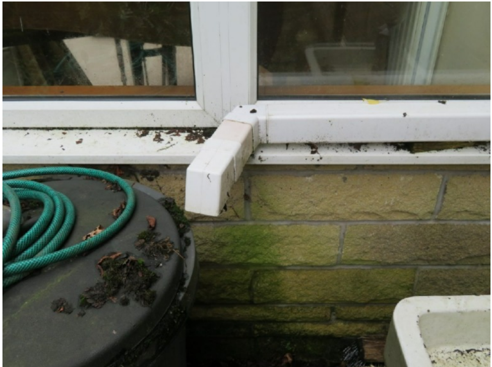
Downpipe from conservatory
