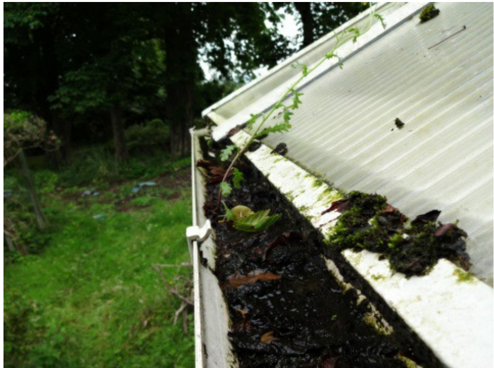
Blocked gutter
