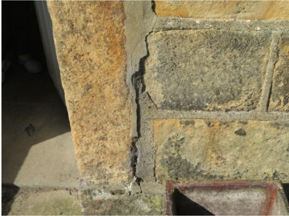
Eroded pointing
