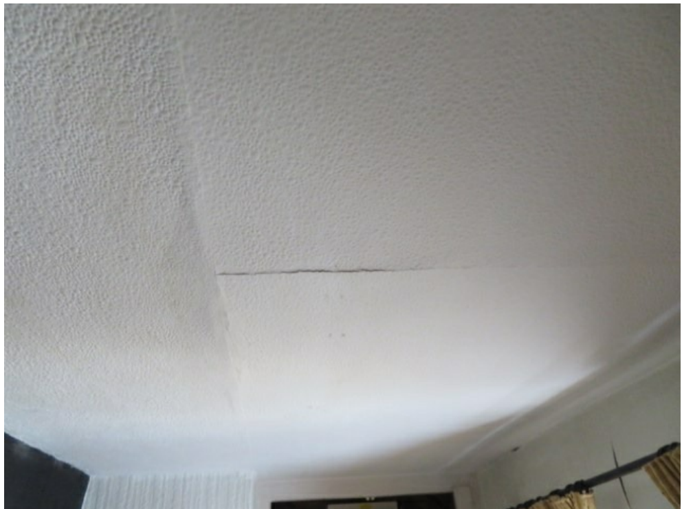
Plasterboard cracks
