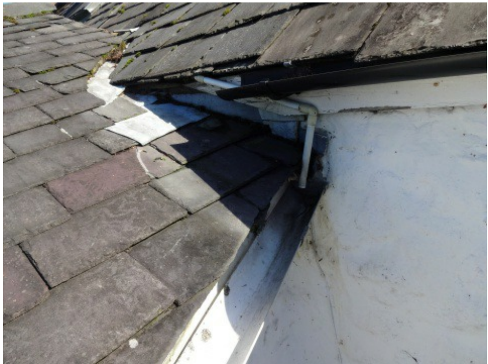
Condensate pipe into gutter
